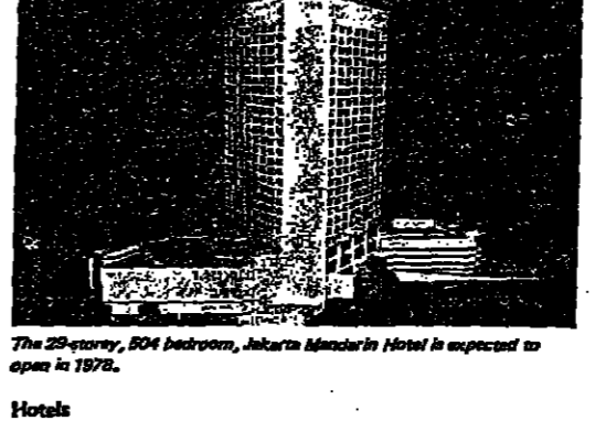
The 25-storey, 504 bedroom, Jakarta Mandarin Hotel is expected to open in 1978.
